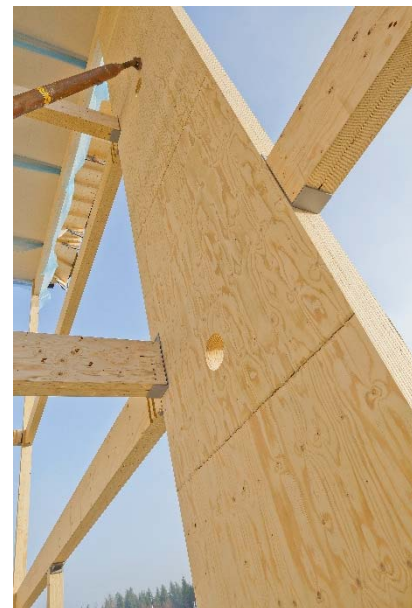
Figure 49: A bracing column made of glued Kerto-Q component.
