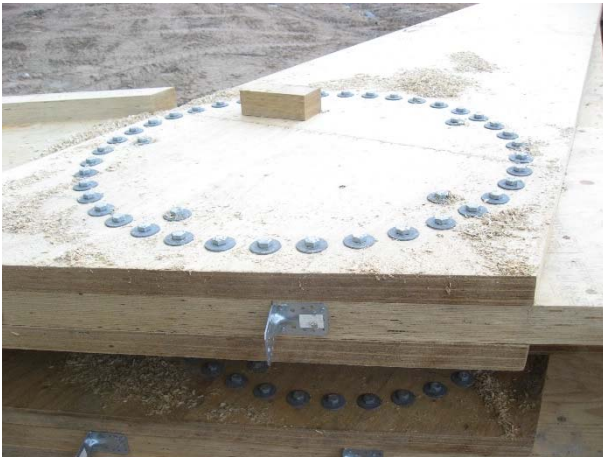
Figure 26: A rafter installed between the Kerto-Q members and connected with bolts.
