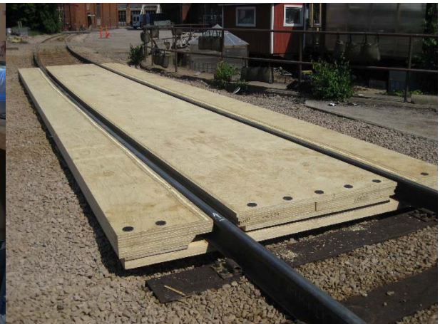
Figure 43: Glued Kerto-Q deck components for railway crossings.
