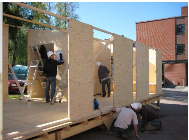
Figure 2: Versatile use of Kerto-Q panels in floors and walls.
