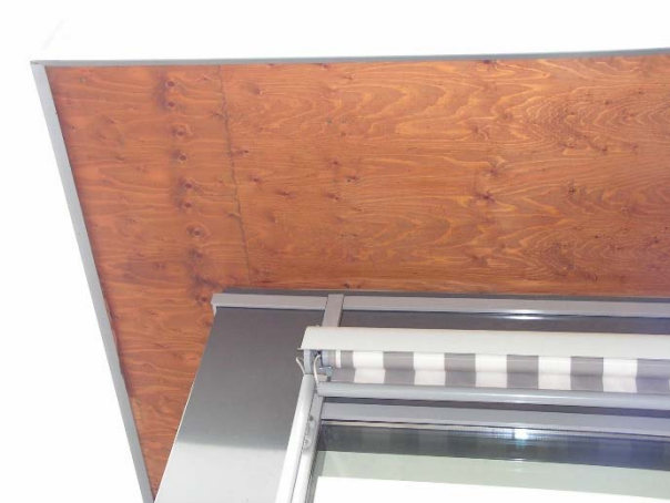
Figure 15: Corner overhang made from Kerto-Q panel.
