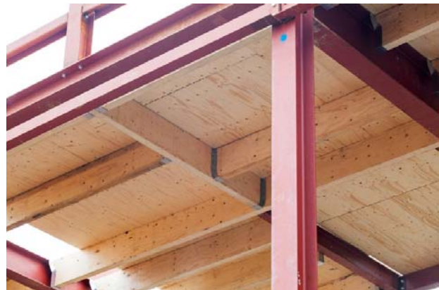
Figure 9: Kerto-Q panels in a roof structure bracing.
