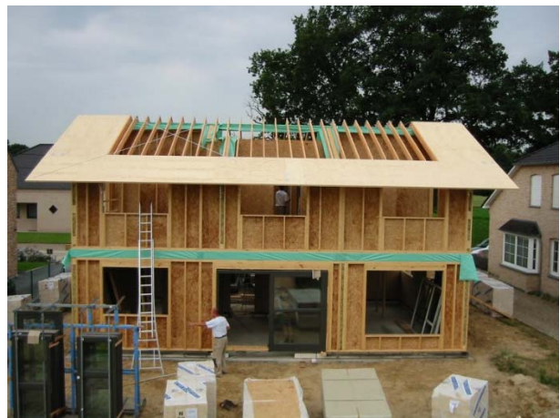
Figure 16: Kerto-Q eave panelling.
