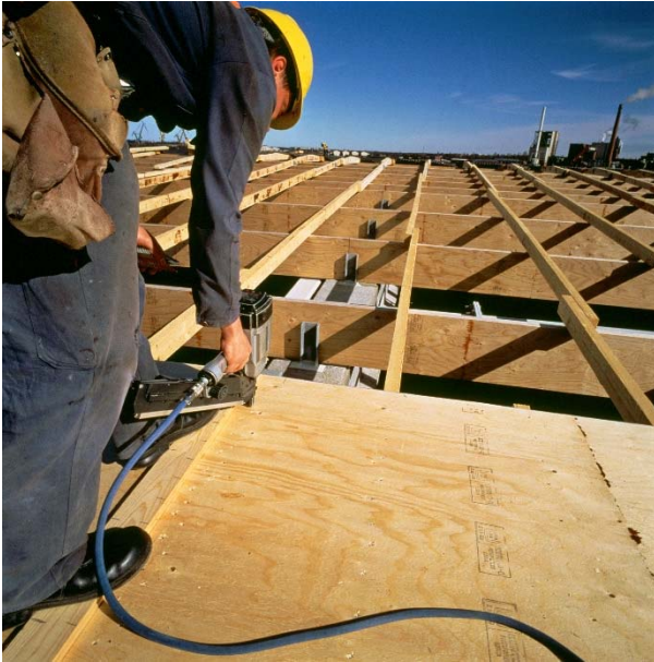
Figure 46: Nailing a Kerto-Q roof panel to the frame. Figure 47: Kerto-Q wall panelling.
