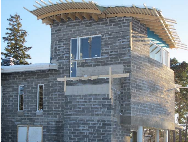
Figure 34: Curved Kerto-Q rafters in a detached house.
