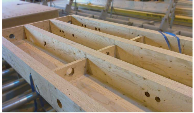
Figure 28: Holes in the beams of a floor element.
