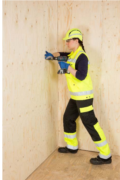
Figure 46: Nailing a Kerto-Q roof panel to the frame. Figure 47: Kerto-Q wall panelling.
